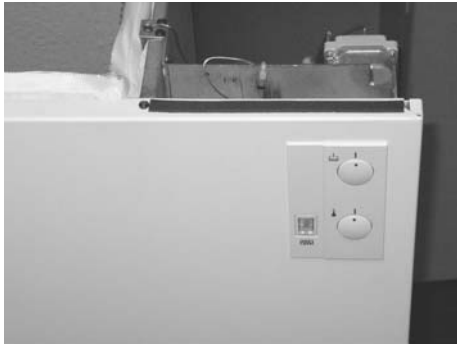
Fig.6 Sealing strip on the front panel edge
