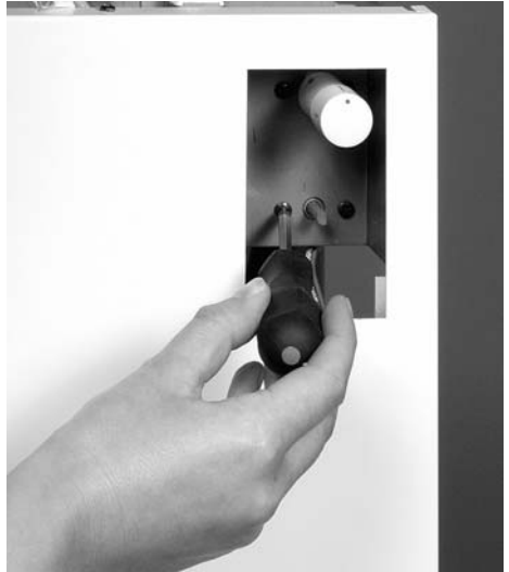
Fig.2 Fixing the capillary-tube thermostat
