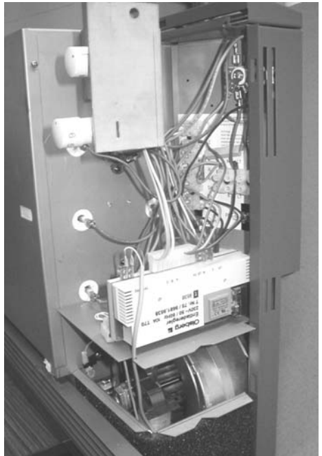
Fig.7 Wired discharge thermostat
