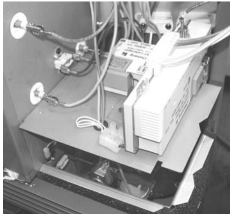
Fig.4 Fixing the discharge thermostat
